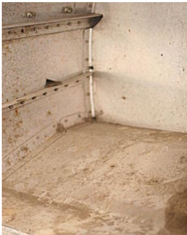
Figure 6-2. Direct chemical attack in a battery compartment.
