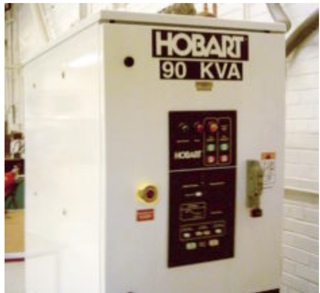
Figure 11-28. A stationary electrical power unit.
