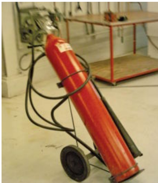
Figure 11-4. Carbon dioxide fire extinguisher.
