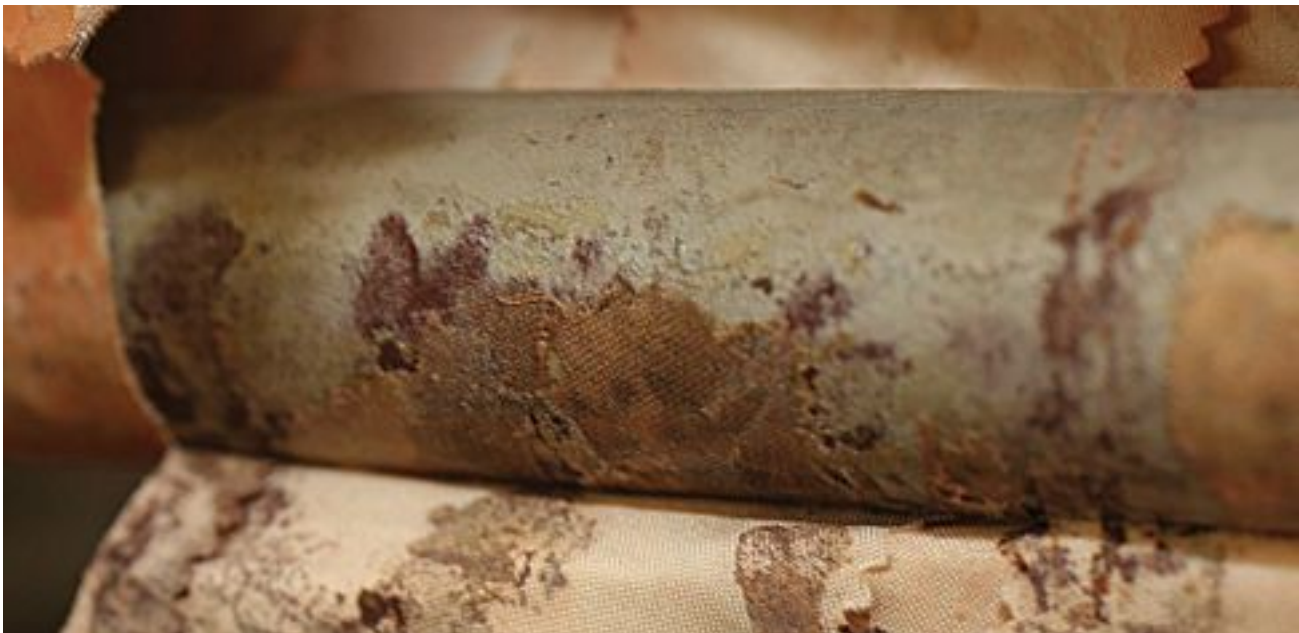
Figure 6-15. Rust on structural components.
